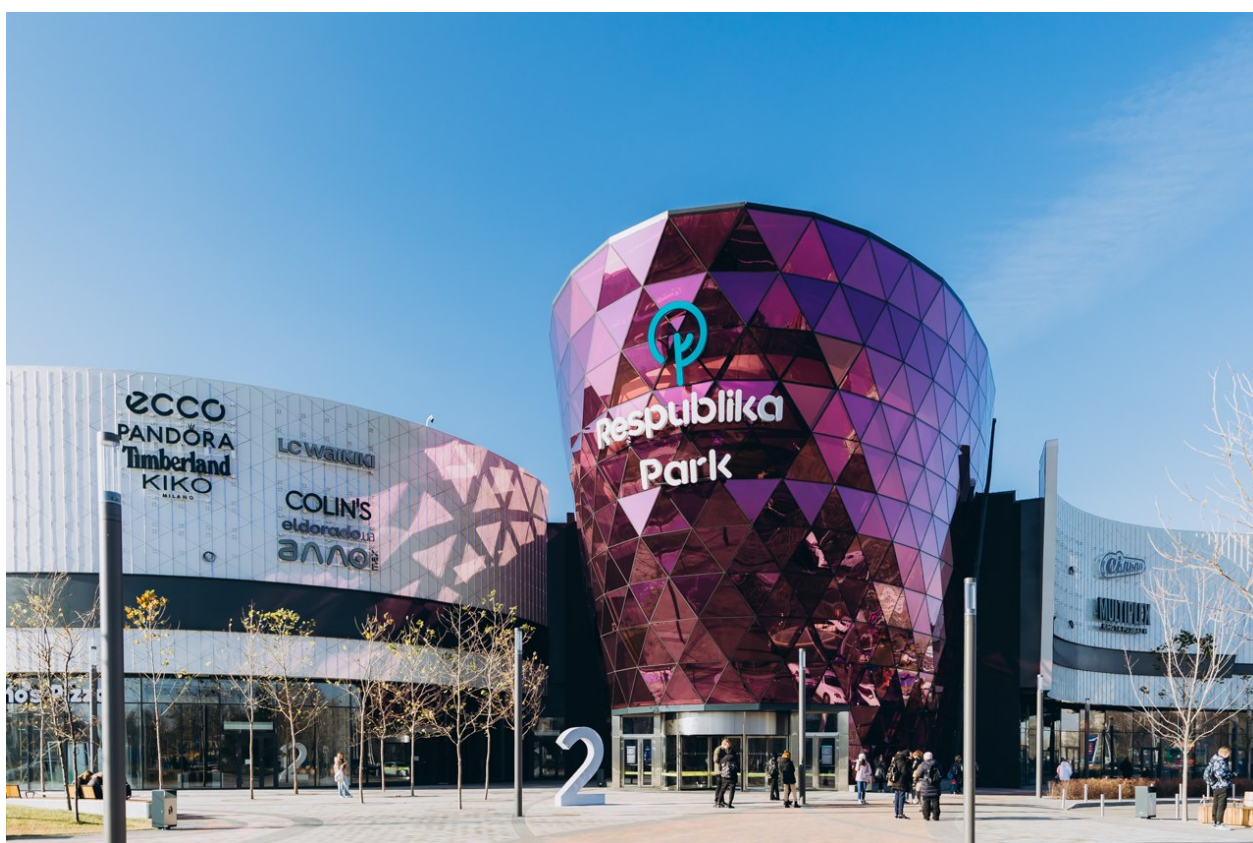
Figure 1 - BIM model and facade of the largest in Ukraine shopping center "Respublika" in Kyiv (arch. bureau "Archimatika", 2014)
