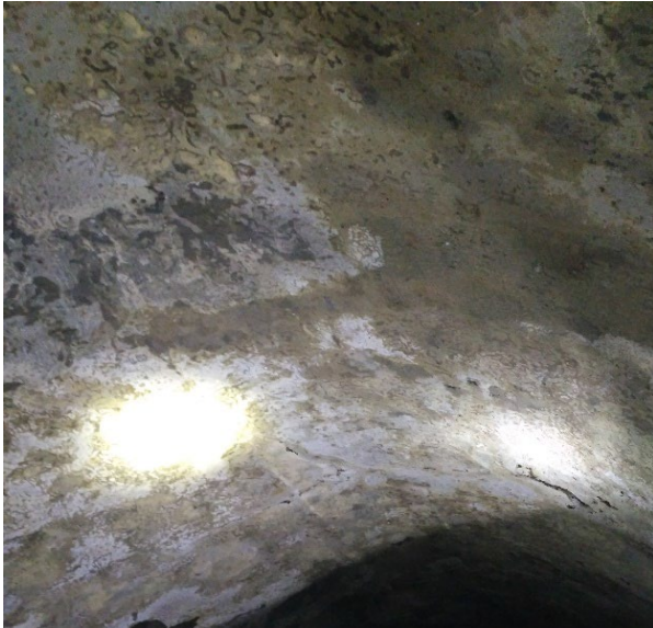
Photo 2 – Vault of the sewer collector
