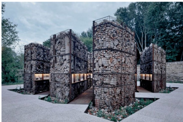
The gravel extracted during the earthworks was used as filler for the gabions. The gabions display the cleaned debris and serve as exhibition structures. The panels contain information about the post-war history of Warsaw and the Czerniaków mound.
